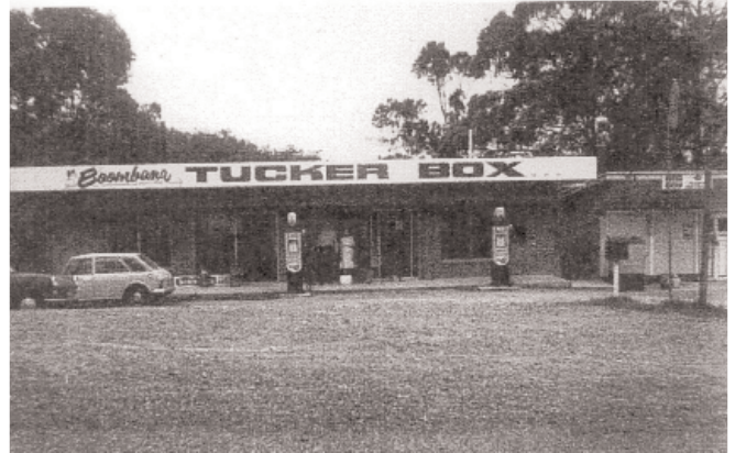
The Cafe Boombana; how it looked in the late 1960s early '70s with 'Tucker Box' written on the fascia. Established by the Bradford family as a Cafe, Shop, Post Office and petrol outlet. Note the fuel bowsers in front, and the word Boombana was also in use at the time.
